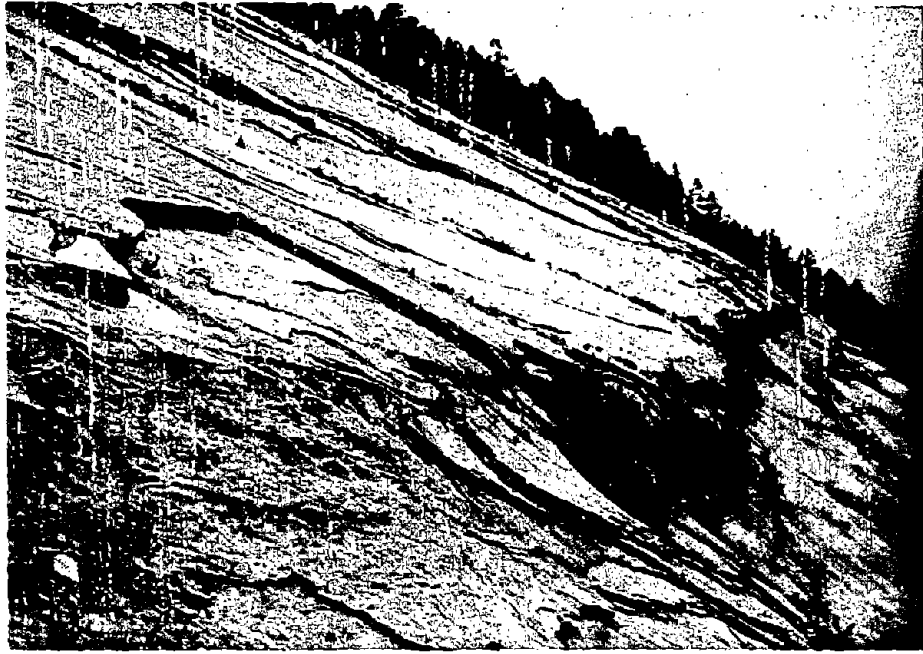
Photo 43. Locations 9-2 and 522-6, middle of western rock face of slide; monocline fold exposed after the 1963 slide is associated with a clay interbed 0.2 to 1 cm thick; bedding dips 36-40^\circ above monocline and 30^\circ below
