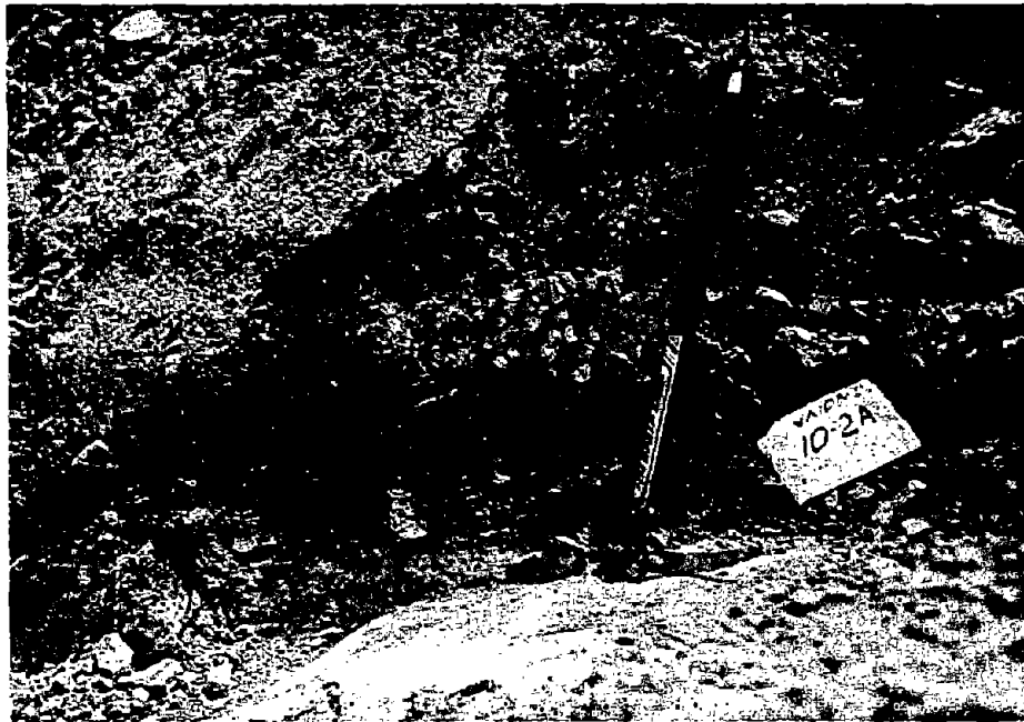
Photo 4. Location 10-2A, base of second gulley from west side of surface of sliding; clay layers 0.5 to 2 cm thick are present in slide debris and along failure surface
