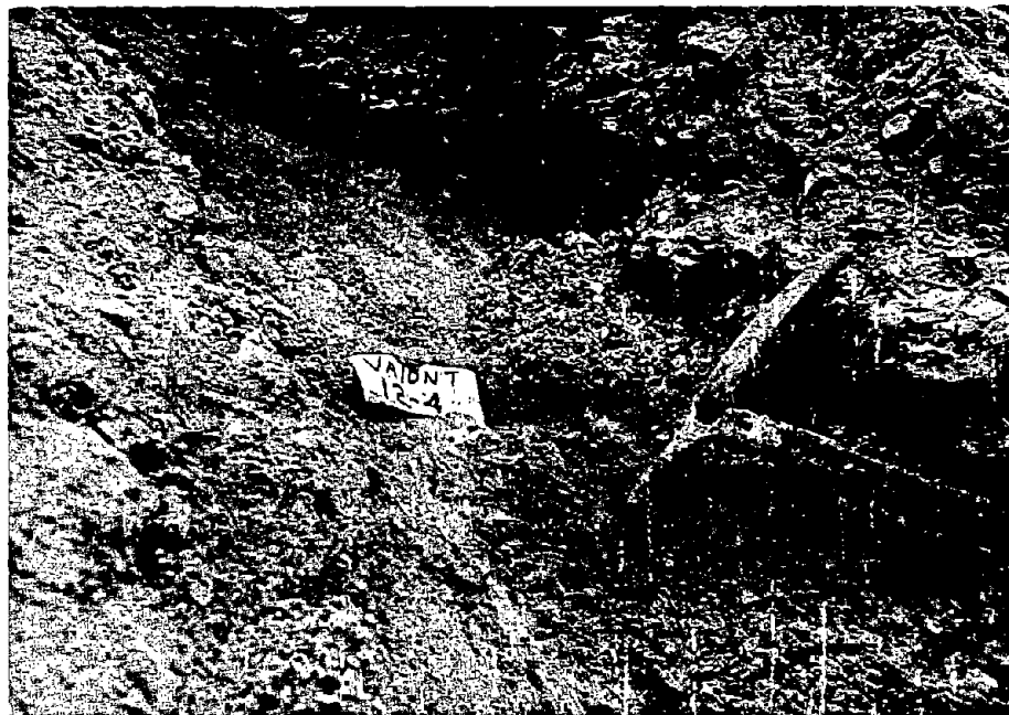
Photo 18. Location 12-4, near east side of slide approximately 70 m above location 12-3; clay layer 0.1 to 1.5 cm thick with a dip of 38° N is present on surface of sliding
