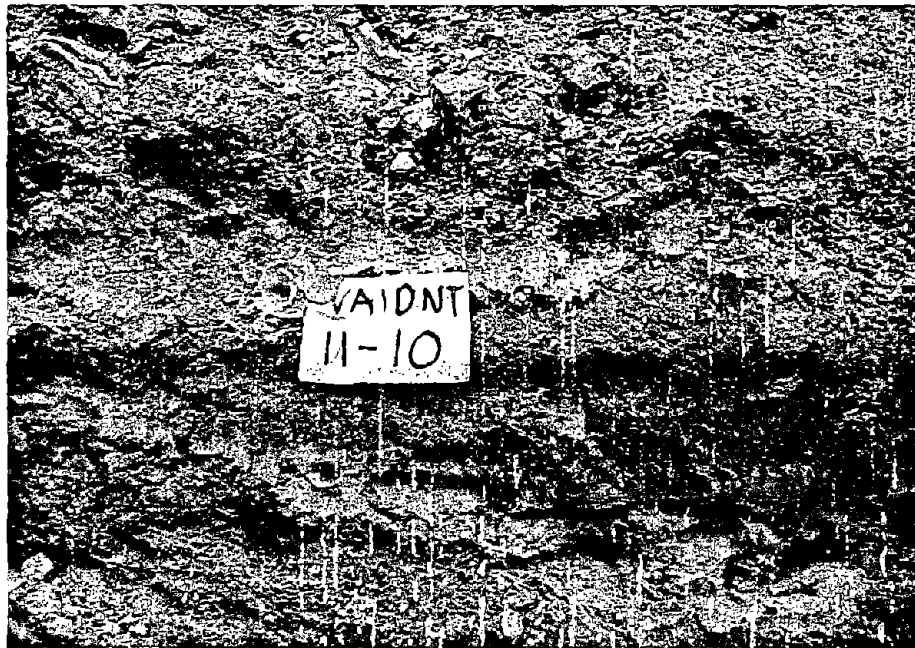
Photo 14. Location 11-10, fourth gully from west side of slide; five layers of clay 1 to 2 cm thick lie in lower 1.5 m of slide debris; failure surface appears in lower left corner
