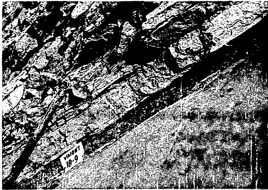
Photo 26. Location 18-9, loose rocks were removed exposing clay interbed 5 cm thick on edge of failure surface; other thin clay interbeds to 0.5 cm maximum are exposed in rock mass above
