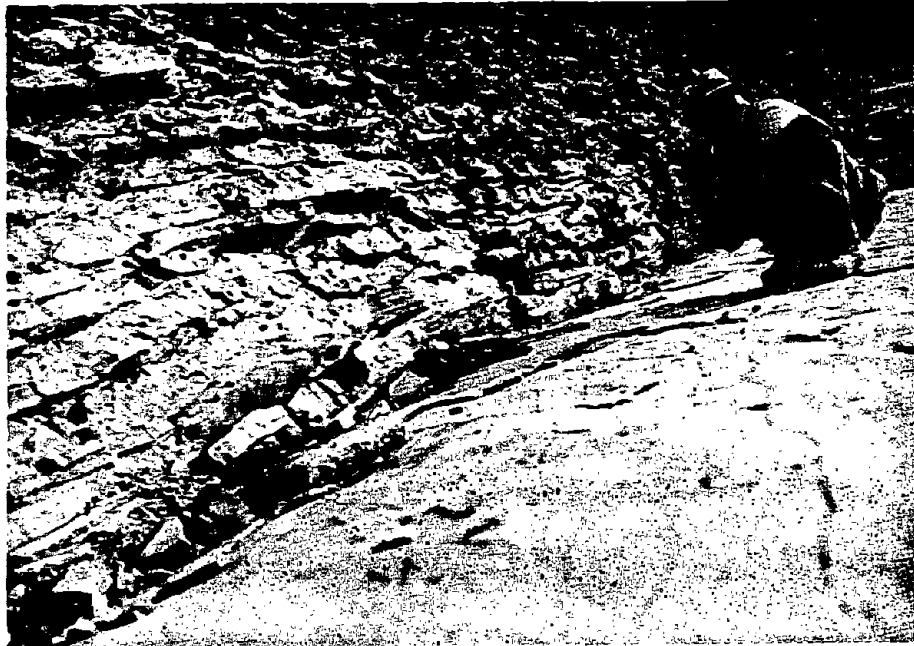
Photo 25. Location 18-9, below western third of headscarp; outcrop along edge of failure surface of 1963 slide or post-1963 slides; loose rock slabs cover clay interbed with dip of 35°N
